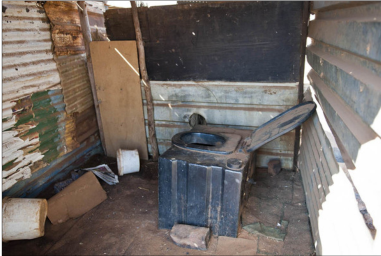
Figure 5: Example of a pit latrine [24].
