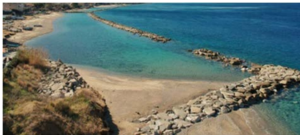
Figure 3: The coastal defence works completed in 2015.
