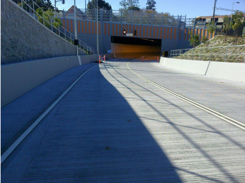
Figure 1: Photo of the as built western portal.
