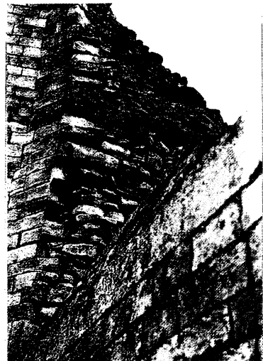
Figure 3: Header stones provided for stability
