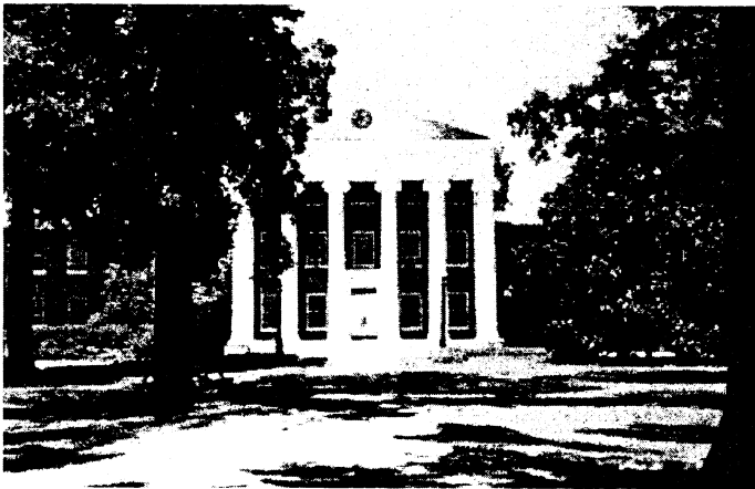
Figure 1. Lyceum building- view from the south.
