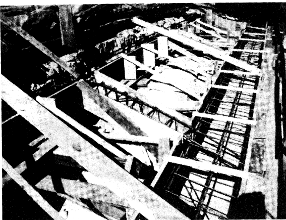
Fig 15.- Construction of hoops
