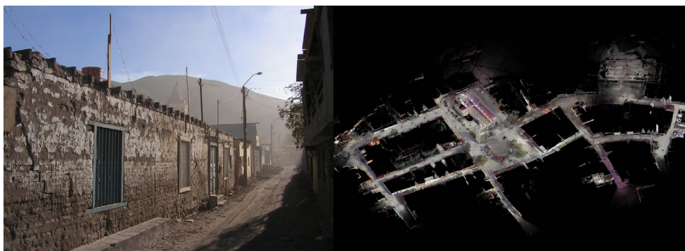
Figure 1: San Lorenzo de Tarapacá-Chile damaged after the 2005 earthquake (left) and after governmental reconstruction from the terrestrial 3D-laser-scanning obtained on-site in 2013 (right). ( Source: Bernadette Devilat. )
