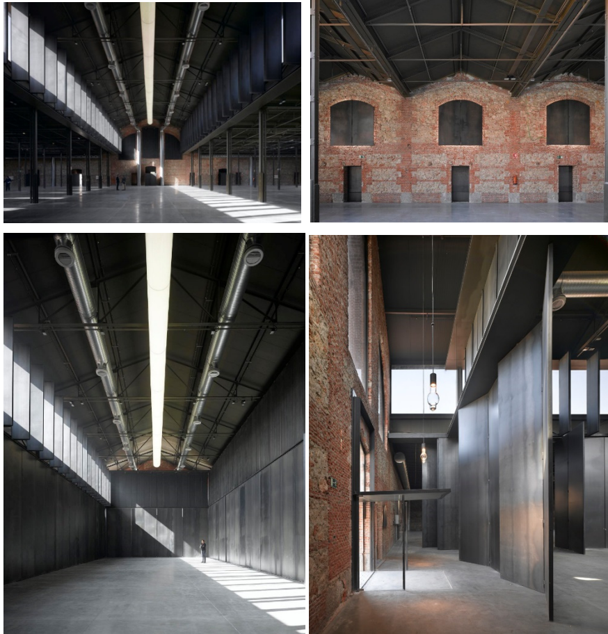
Figure 17: Interior views of the current state of pavilion 16.
