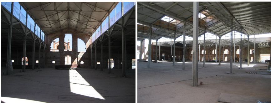
Figure 7: Interior views of the original state of pavilions 15 and 16.
