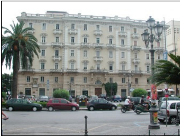
Figure 1: Picture of the north façade.
