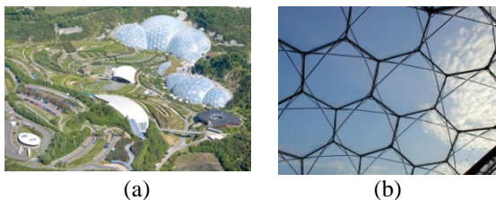
Figure 5: Eden project to the left the panoramic view of the geodesic biome domes, to the right the hex angle structure [9].
