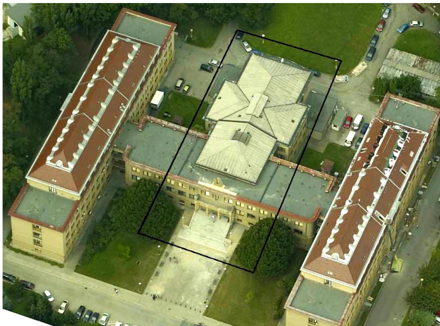
Figure 1: General view of the university complex.
