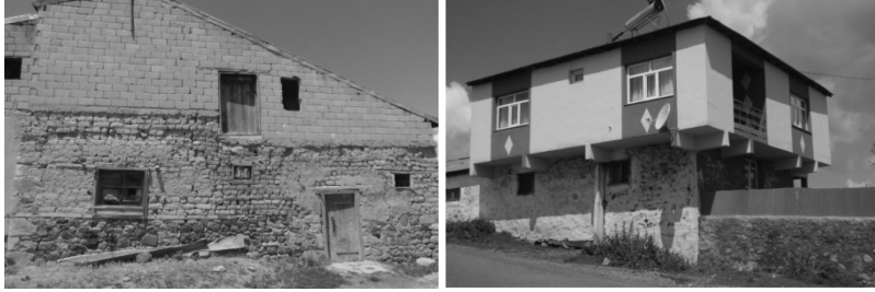
Figure 10: The exterior view of hybrid houses, which were added the second floor with non-local materials, while the walls in ground floor were local materials, samples from Erzurum, on the left, and Ardahan, on the right (photos taken by the author).
