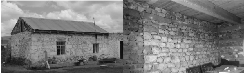
Figure 7: The exterior view of a maintained house with rubble stone wall, on the left; the interior view of a renewed rubble stone wall, on the right (photos taken by the author).
