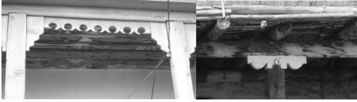
Figure 5: The examples of woodworks applied to the post-head for terrace roof (photos taken by the author).
