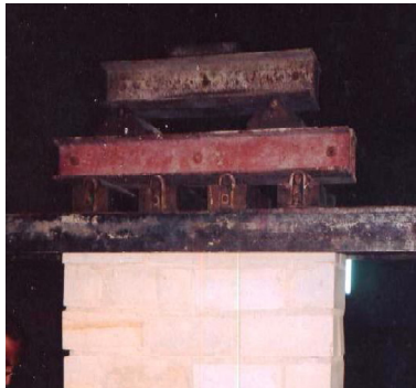
Figure 3: Loading beam on wall top.
