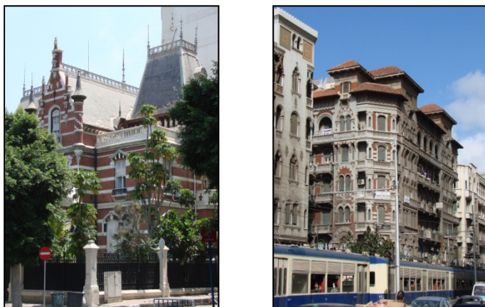
Figure 1: Examples from the architectural heritage of Alexandria.
