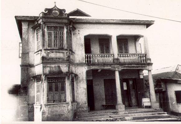
Figure 7: Ologbenla House, before the intervention. Note the chipped steps, missing balusters and general shabbiness.
