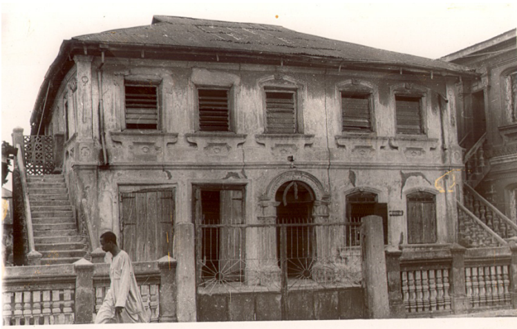
Figure 2: Olayinka House, before the tentative restoration, faded and cracked.
