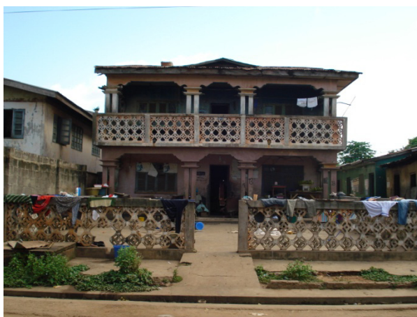
Figure 4: Ile Alubarika . Approach façade. Looking deceptively well-kept even at the time of the intervention, the house was in very bad shape.
