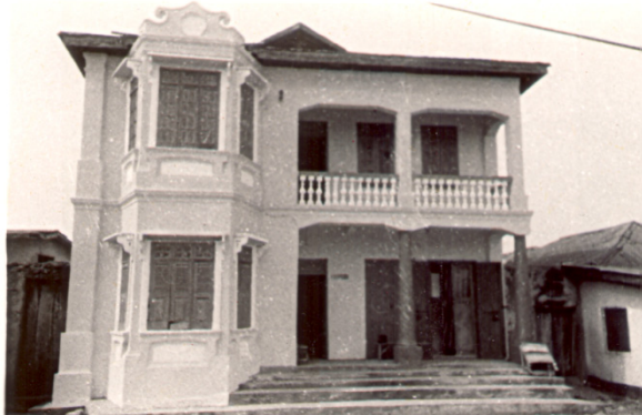
Figure 8: Ologbenla House, after, sporting a new coat of paint and repaired steps. The baluster replacements (4 th & 5 th left) could not be exactly matched.
