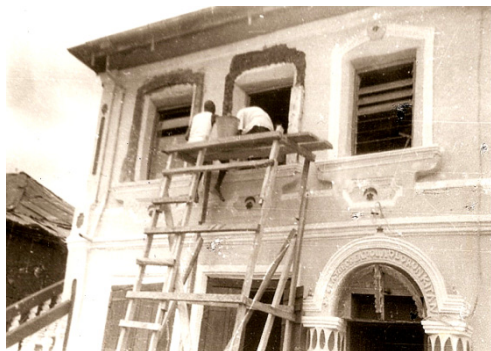
Figure 3: Restoration of decorative moulding around upper windows.
