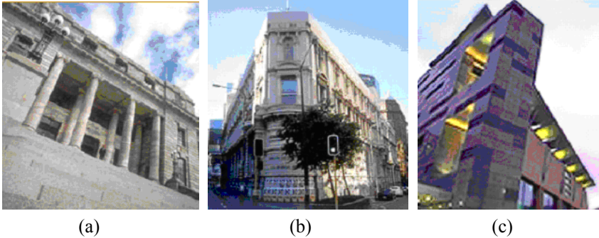
Figure 5: Base isolated structures in New Zealand: (a) Parliament building, (b) Old bank in Wellington, (c) the Museum of New Zealand.
