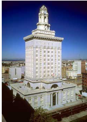
Figure 3: Base isolated Oakland City Hall.
