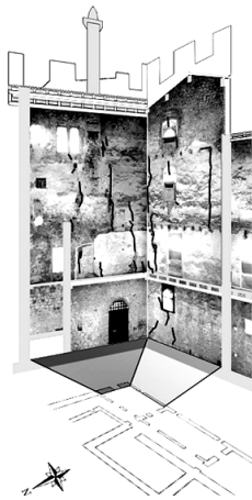
Figure 3: Crack pattern of the Tower.
