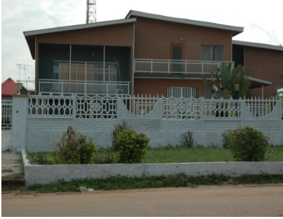
Figure 13: Balustrades in “modern” materials: glass-and-aluminium balustrades, with factory-produced panels as fencing, Ondo.
