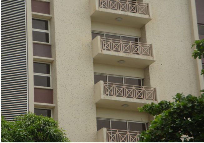
Figure 6: High-rise multi-apartment building, Ikoyi, Lagos, March, 2010; yet to be let. Balconies feature the colonial balustrade motif, adapted.
