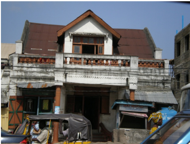
Figure 2: Second-generation Afro-Brazilian house ca. 1960; Yaba, Lagos. Squat, bulbous concrete balusters are used in the balcony.
