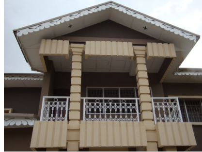
Figure 14: Balustrades in “modern” materials: metal balustrade using galvanized pipes and reinforcement iron, Ile-Ife.
