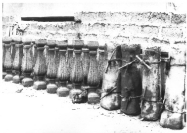
Figures 19: Bulbous balusters, exposed and some still in moulds (right).
