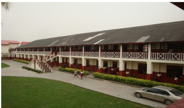
Figure 5: Holy Child College , Lagos; built in 1945. First school block. Skeletal concrete panel, with 'X' motif.
