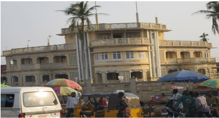
Figure 4: Goodwill Lodge (Okunnowo house), Ijebu-Ode was built in the early 1960s; it is copiously balustraded with perforated panels.
