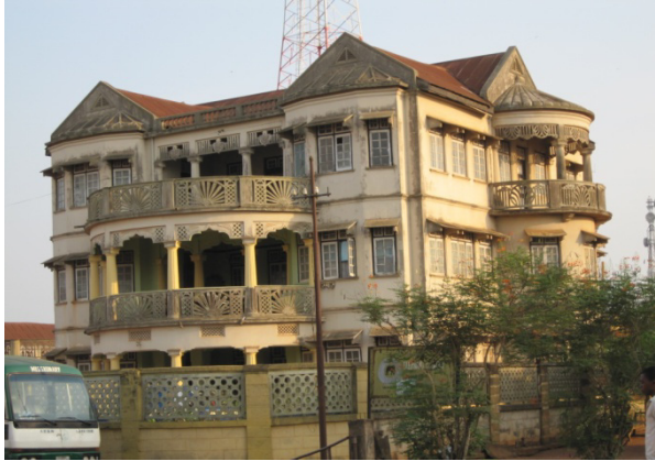
Figure 3: Kekere-Owo house, Ijebu-Ode. Built in the 1940s, it features concrete panel balustrades (and fretwork), but also has balusters at roof level.
