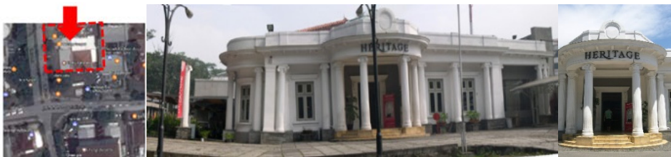
Figure 4: The location and front elevation of the "Heritage" factory outlet building. (Source: Edited from Google maps, 2018 and Nurtati Soewarno, 2005.)
