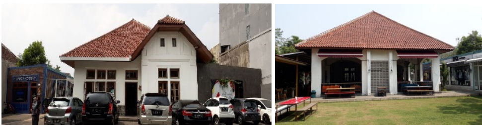
Figure 11: Current front and back yard elevation. (Source: Survey result, 2018.)
