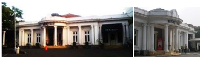
Figure 2: The first building in Riau Street 63 was an official residence of the Director of Government Companies. (Source: Katam, 2010.)
