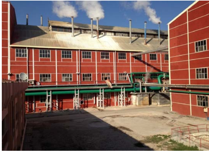
Figure 7: Sugar Factory buildings constructed with steel and local brick. (Source: Photographed by the author.)
