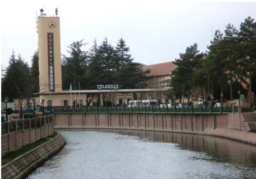
Figure 5: Tülomsaş, Eskişehir Railway Factory lies in between the Porsuk River and the railway at the city center. (Source: Photographed by the author.)
