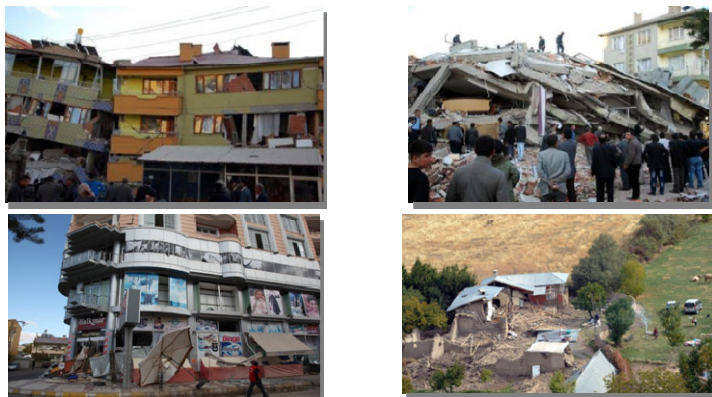
Figure 4: Photos showing destroyed and damaged urban and rural buildings.
