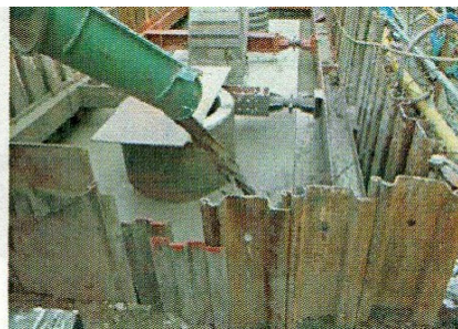
Figure 9: Pouring fluidization soil directly from the transit mixer.
