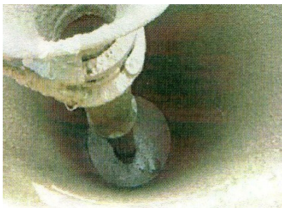
Figure 8: Pouring fluidization process soil using a tremie pipe.
