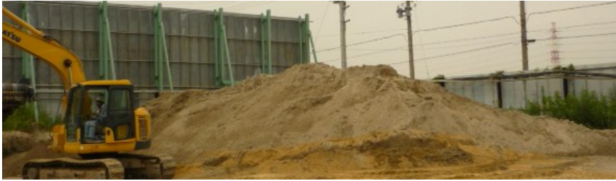
Figure 5: Recycled natural sand.
