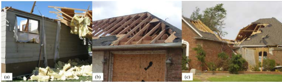
Figure 1: Residential (FR12) roof failure modes. (a) Roof-to-wall connection (RTWC) failure; (b) Sheathing loss; (c) Framing failure. (Source: Authors and Dr. D.O. Prevatt, University of Florida.)
