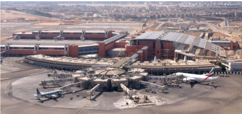
Figure 1: TB2 (foreground) and TB3 (background).
