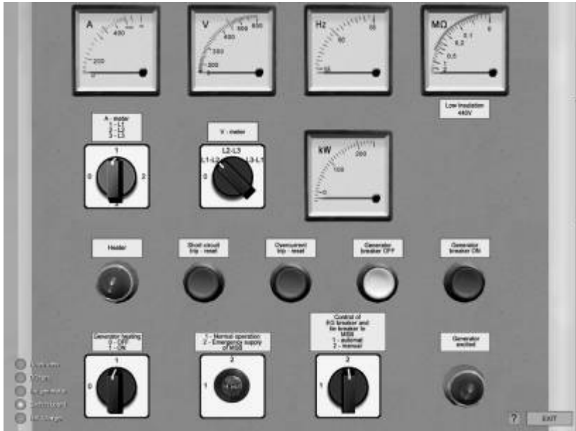
Figure 9: Zoomed emergency switchboard control panel.
