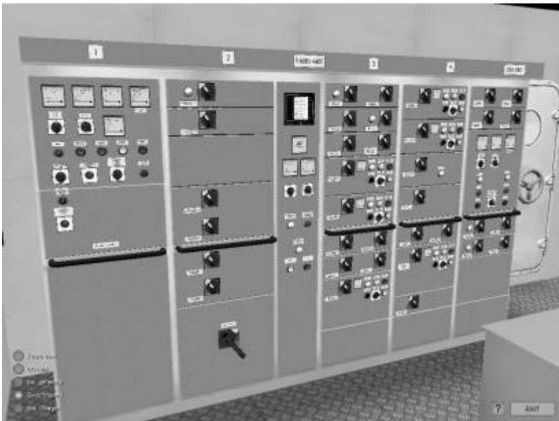
Figure 8: Emergency switchboard – general view with zoom selections.
