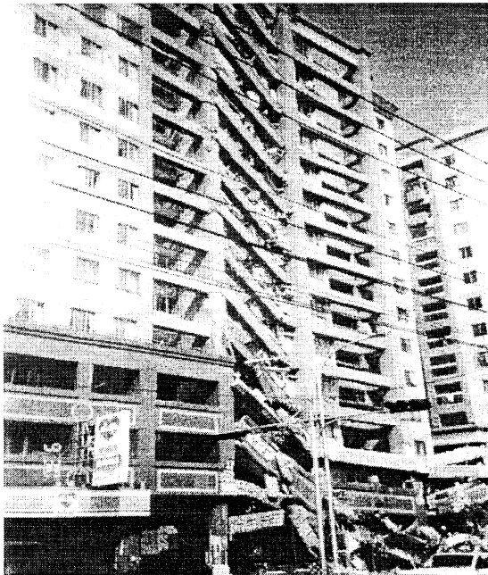
Figure 10: Representative types of collapsed mid-rise buildings.
