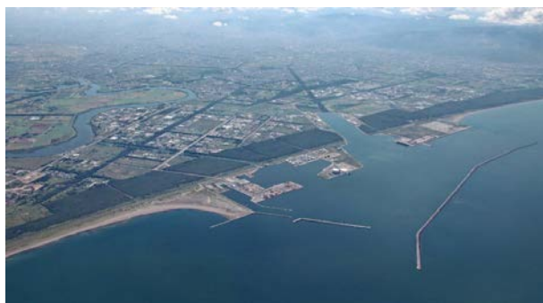
Figure 10: Aerial view of Ishikari Bay new port.
