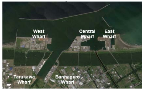
Figure 11: Facilities of the Ishikari Bay new port.
