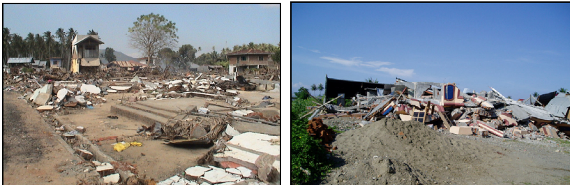
Figure 6: Poor seismic performance of domestic buildings in Aceh.
