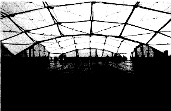
Internal view of swimming-pool.
