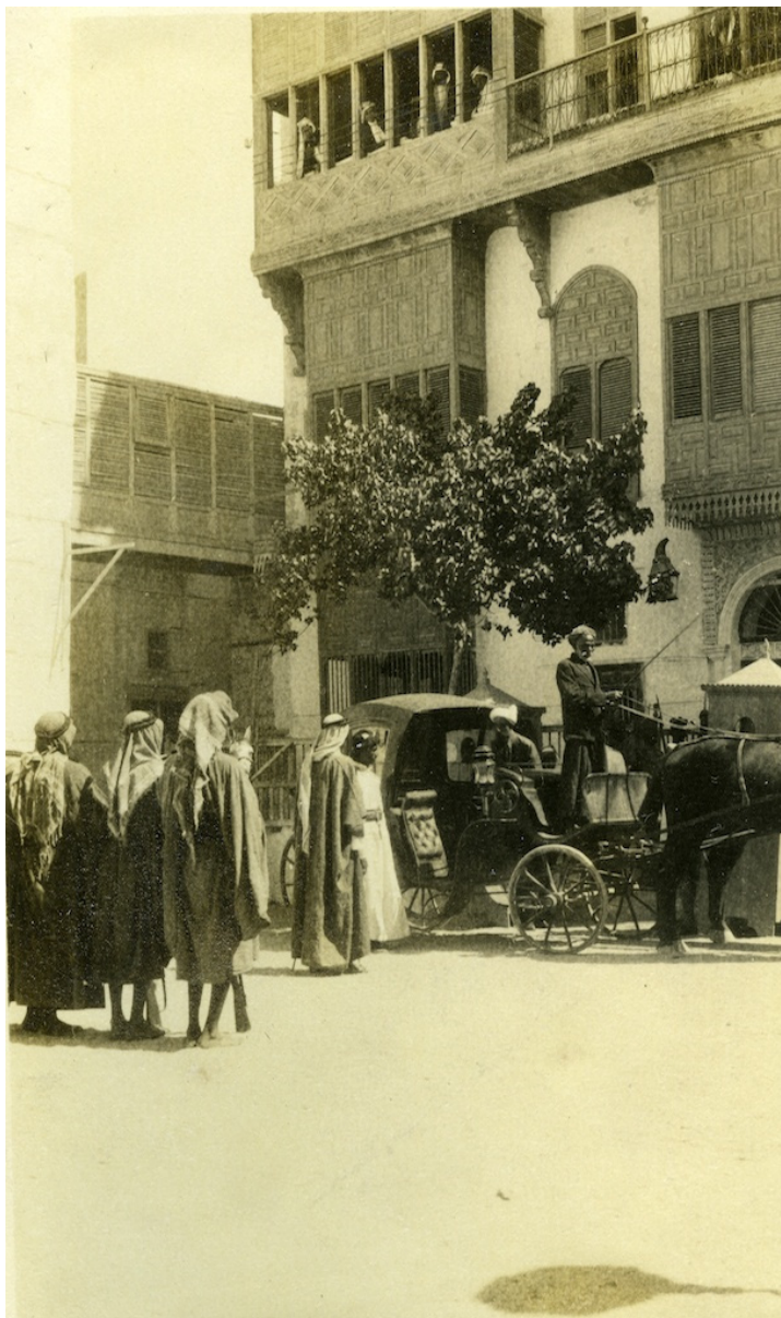
Figure 4: Al Sharif Taha Mhana House taken by St John Philby 1925. (Source: http://lostopportunitiesandwastedtimes.blogspot.com/2014/07/blog-post_25.html .)
