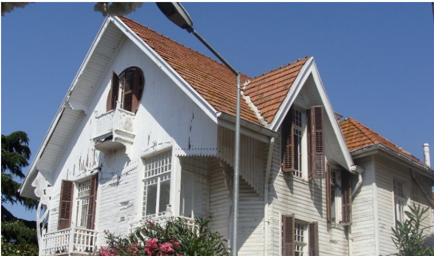
Figure 4: Steeply pitched roof example from Buyukada.
