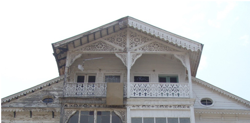
Figure 7: Timber double house with ornaments.
