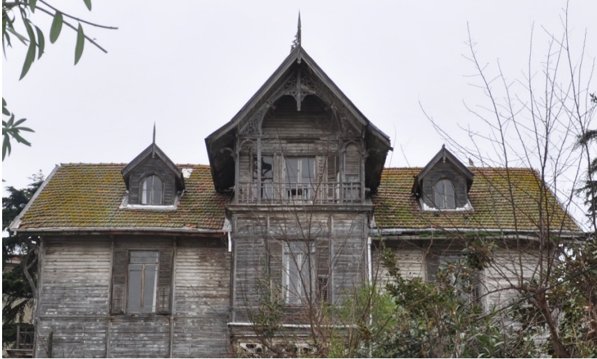
Figure 8: Roof windows and ornaments of a timber house in Buyukada.
