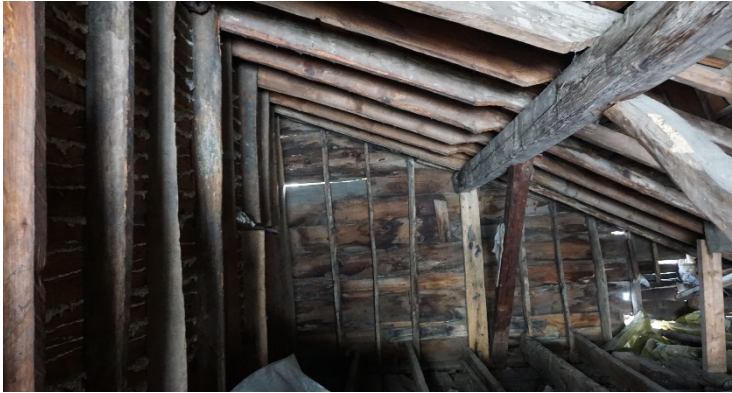
Figure 10: Inner sight of a timber house with ornamented roof.
