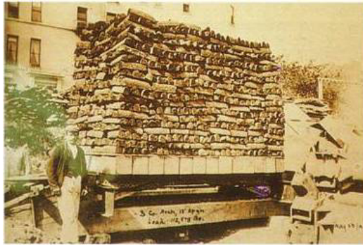
Figure 2: Resistance test affected by Guastavino on a thin vault.
