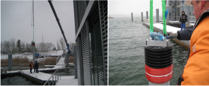
Figure 8: Installation of the heat pipe by means of crane work.
