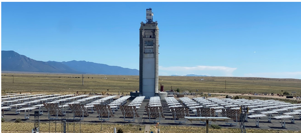
Figure 1: Heliostat field and central solar tower at Sandia NSTTF with solid particle receiver mounted on top of the tower.
