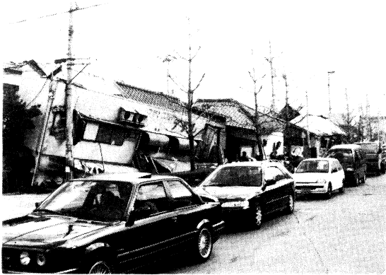
Figure 6. Destroyed wooden houses in Kobe.
