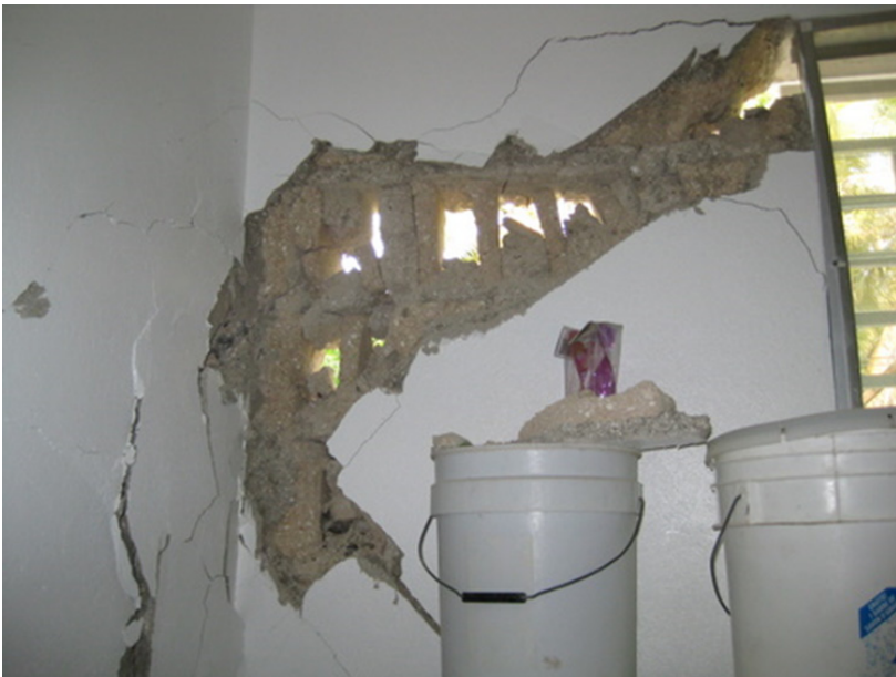
Figure 4: Newly constructed building with a hybrid system of reinforced concrete with CMU block.
