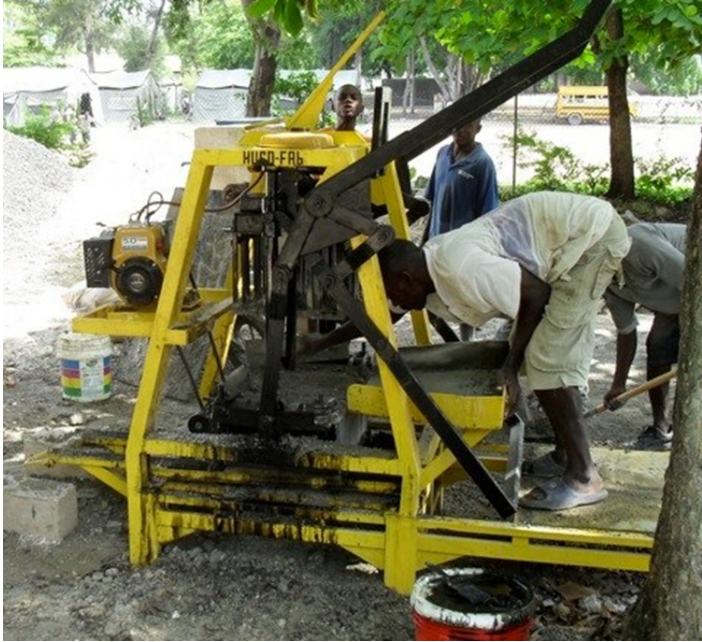
Figure 5: Machine used to make CMU block in Haiti.
