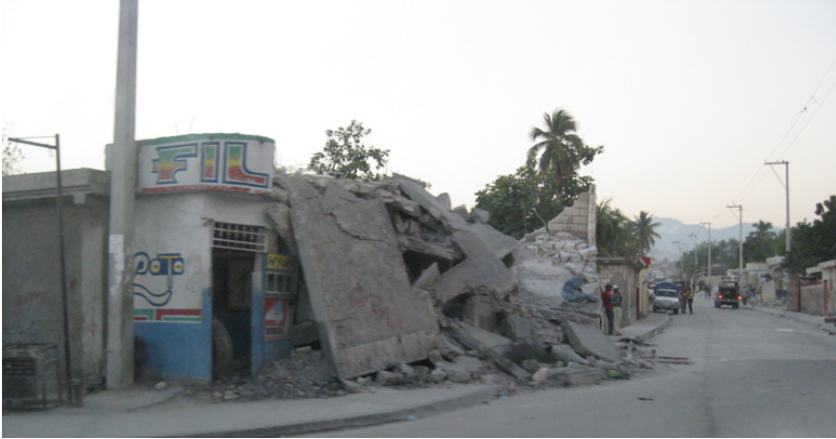
Figure 1: Typical buildings in Port-au-Prince, Haiti shown following the earthquake.
