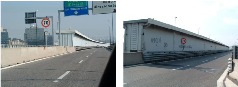
Figure 5: Views of the deck and the main girder.
