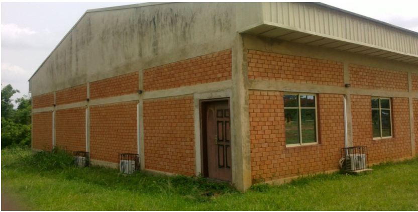
Figure 2: The Electronic Testing Centre of the Federal University of Technology, Akure, Nigeria built with stabilized earth bricks.
