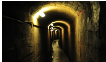
Figure 8: Qionglin civil defence tunnel.
