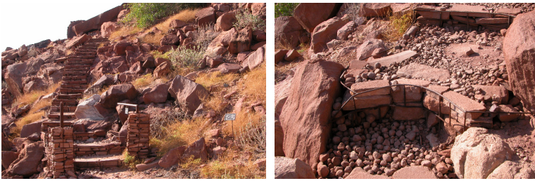
Figure 2: Stone gabions and wire cages, Twyfelfontein, Namibia.
