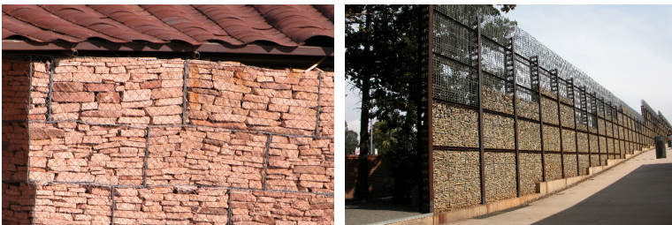
Figure 3: Gabions filled with loose stones and rubble, Namibia and RSA.
