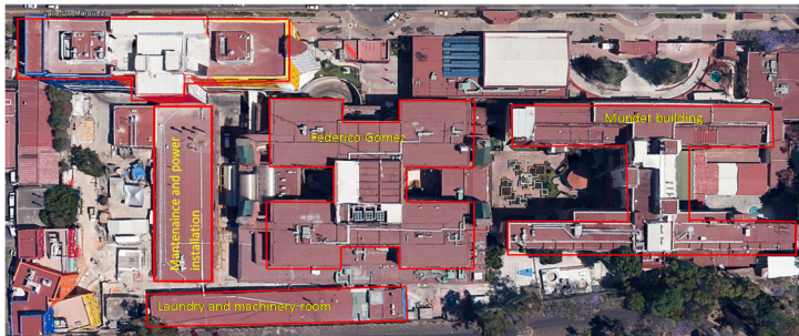
Figure 1: Architectural shape with probability of very high damage to ChH.
