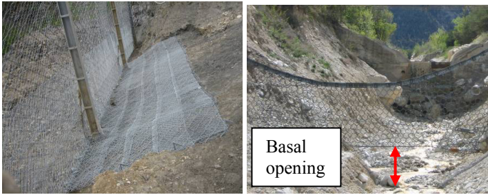
Figure 9: Particular ground adaptation with a fixed mesh for shallow landslide barriers (left) and extra projected basal openings for debris flow barriers (right).
