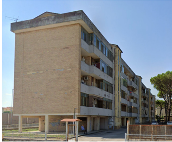
Figure 5: Parasitic volumetric additions in the district “le fornaci” in S. Maria Capua Vetere (CE) Italy: State of fact [9].
