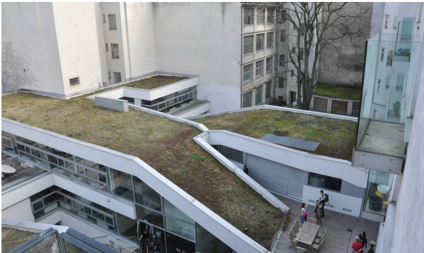
Figure 2: Wimberggasse Townhouse, Delugan and Meissl, Vienna, 2001, (photo: P. Haupt, 2011).
