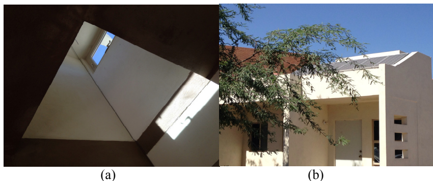
Figure 2: (a) Solar “chimney” and (b) photovoltaic panels on the south façade.
