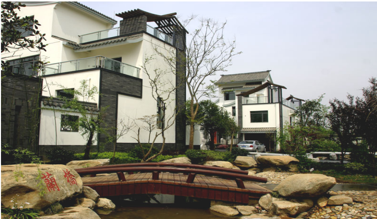
Figure 3: Good combination of Qi of different locally sourced materials in a newly developed residential area in city of Wuhan, central China.
