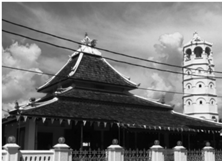
Figure 11: Corrugated ridge roof.
