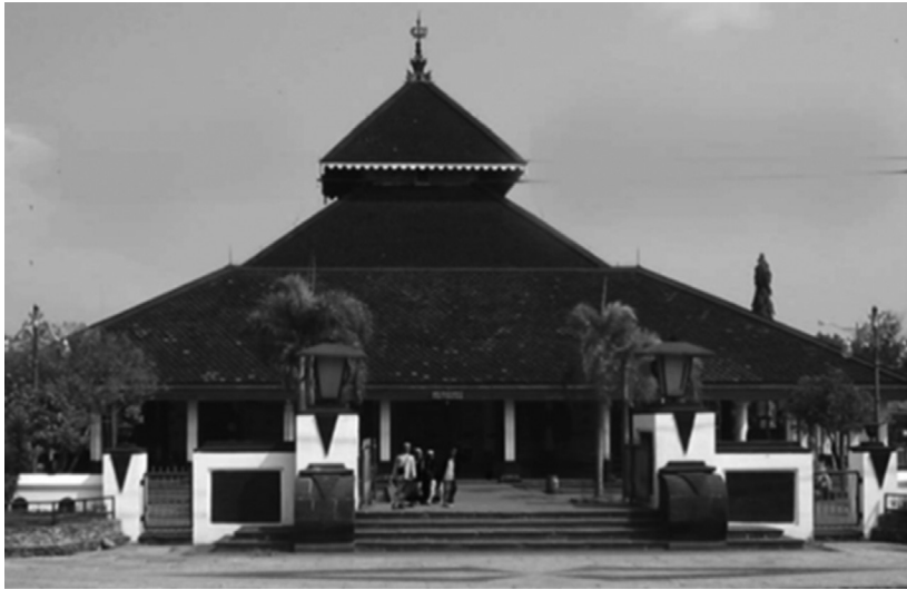
Figure 4: Demak Great Mosque, Indonesia [21].
