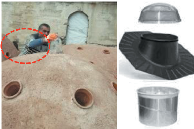
Figure 3: Oculi (light holes) on the vaults/domes of the bath section in Süleymaniye Hospital (left) (photo: archives of Fatma Usluer, 2011) and the light-collecting glass application of today's technology (right) [10].
