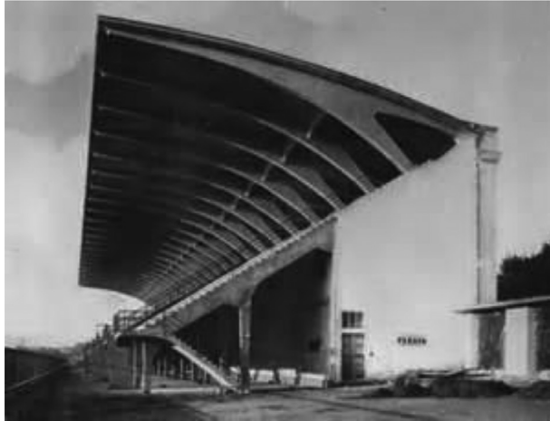
Figure 11: The cantilevered roof of the Municipal Stadium in Florence. Pier Luigi Nervi, 1930–1932 (Source: Nervi [23]).
