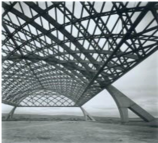
Figure 13: Geodetic structure of the hangars for the Italian air force. Pier Luigi Nervi, 1935–1940 (Source: Nervi [23]).
