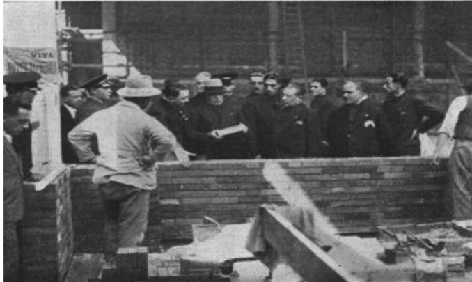
Figure 7: Visit of Mussolini during the construction of load-bearing walls of the Palace of the Art with Litoceramica Italklinker.
