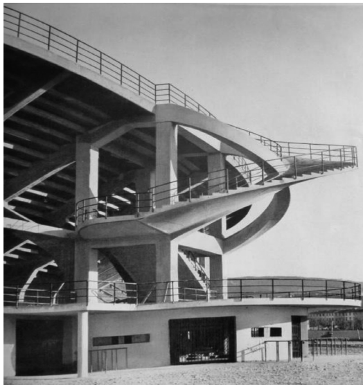
Figure 12: The spiral exterior stairs of Municipal Stadium in Florence. Pier Luigi Nervi, 1930–1932 (Source: Nervi [23]).
