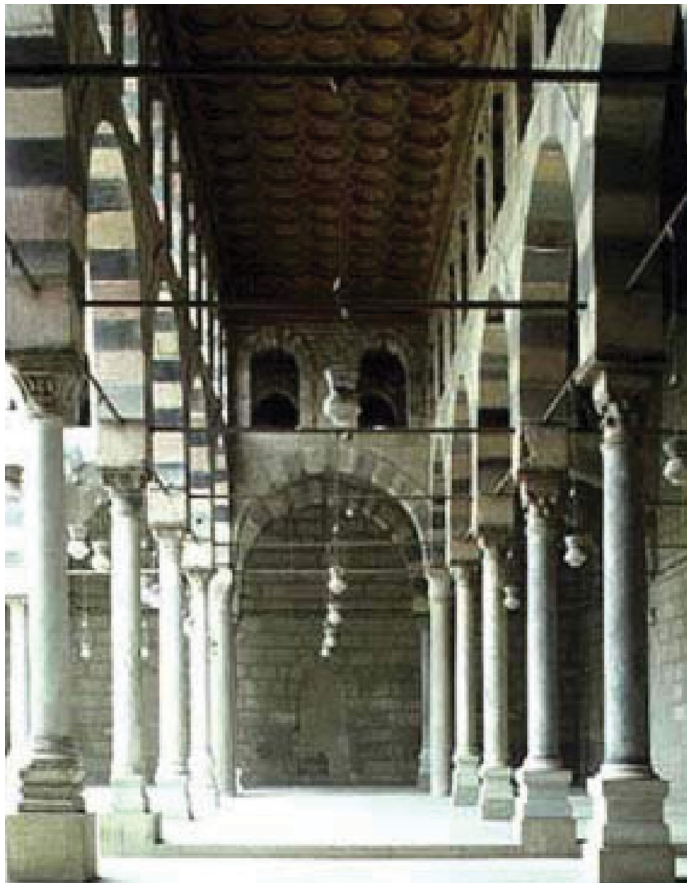
Figure 12: The inside columns in the Al-Nasir Ibn Qalwon Mosque.
