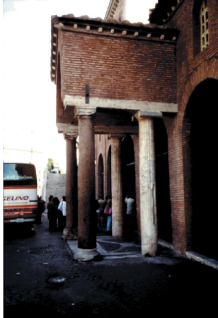
Figure 2: Church of Santa Maria in Cosmedin, Rome – The porch portal of the church, two different Ionic columns, white marble and red granite [6].
